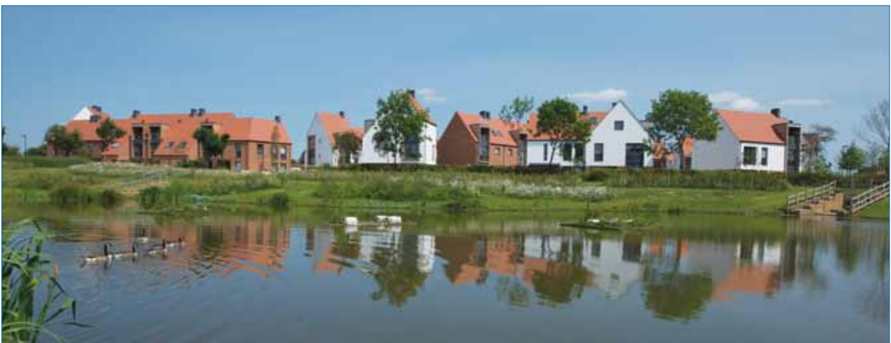
Derwenthorpe housing development
